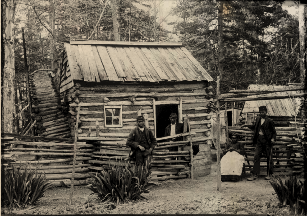
Above The early slave house on Mason Barkley's plantation may have looked very much like this Bon Air, Virginia example photographed in 1888. Typical of slave houses, the small log structure shown here has a wooden roof of long boards rather than a fully shingled roof, a small window, and a leaning stick and mud chimney propped-up by poles.
